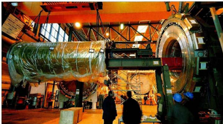
The ATLAS superconducting solenoid during one of the transport operations. Securely attached to the overhead crane, the solenoid is situated in front of the opening to the liquid-argon electromagnetic calorimeter, where it will soon be inserted.
