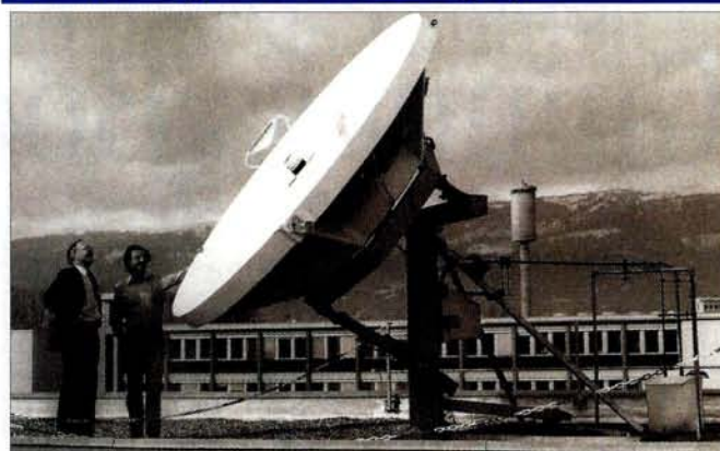
The 3 m diameter antenna that was installed at CERN for data transmission via the OTS satellite in the STELLA project.
